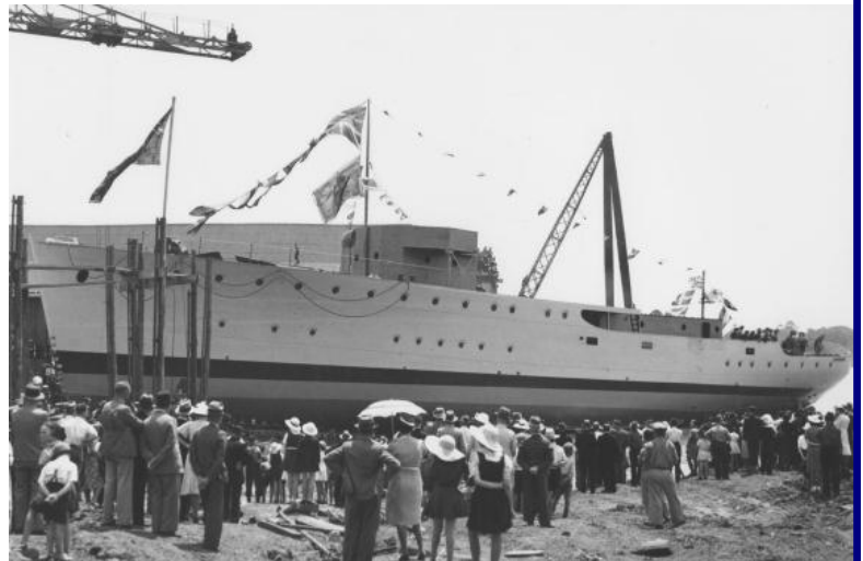
Maryborough sliding down the slipway with bunting flying as workers look on.
